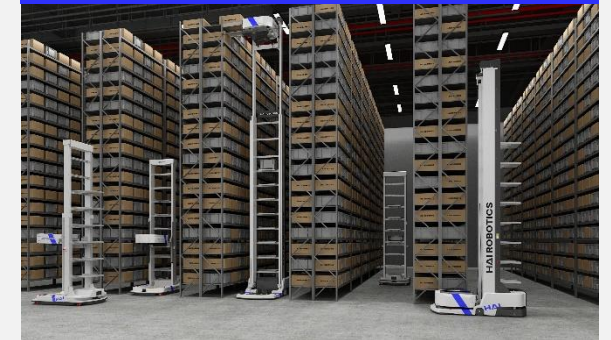
Warehouse 4.0 ACR automated warehouse
