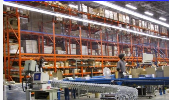
Warehouse 3.0 ASRS automated warehouse
